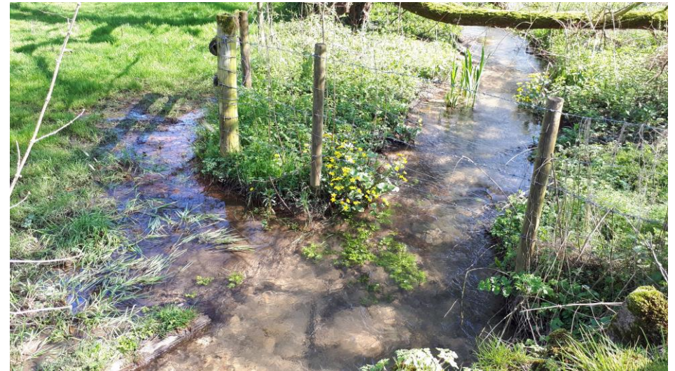
42_looking N US showing pooling and break of R bank_190418
