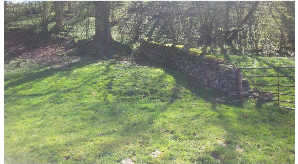
G26_minor seepage on slope facing S
