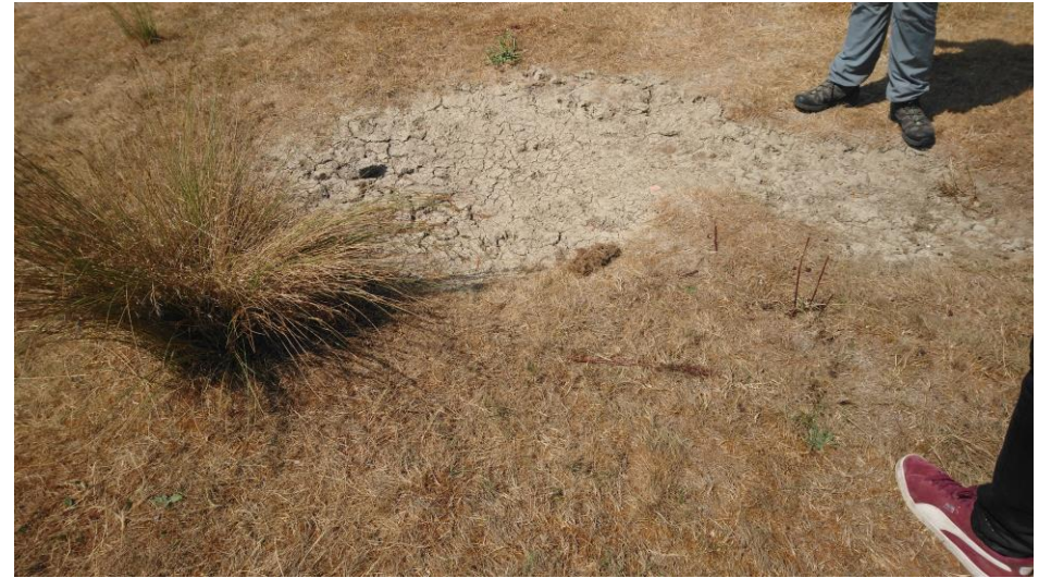
G116_dry seepage patch
