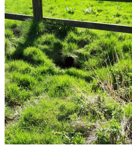
45_looking SE outfall into area marked as pond on OS maps
