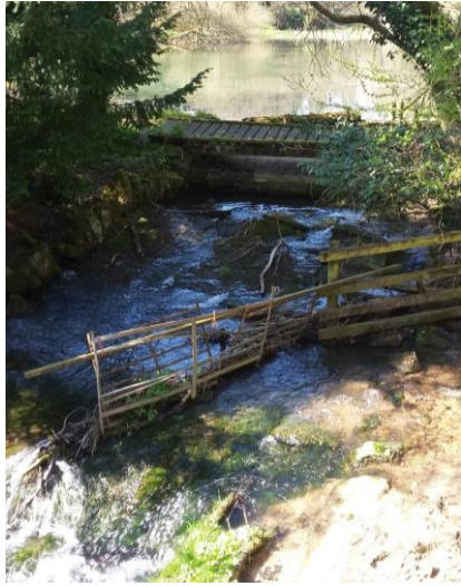
G50_River Churn culverted under road facing NW
