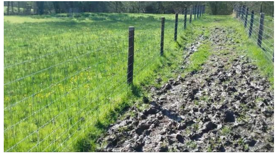
G39_seepage upgradient of River Churn trib starts facing S
