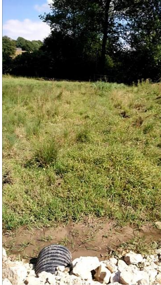
G106_culverted spring fed watercourse facing W
