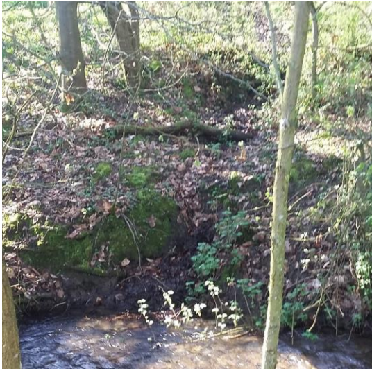
G37_seepage on banks of River Churn trib facing S
