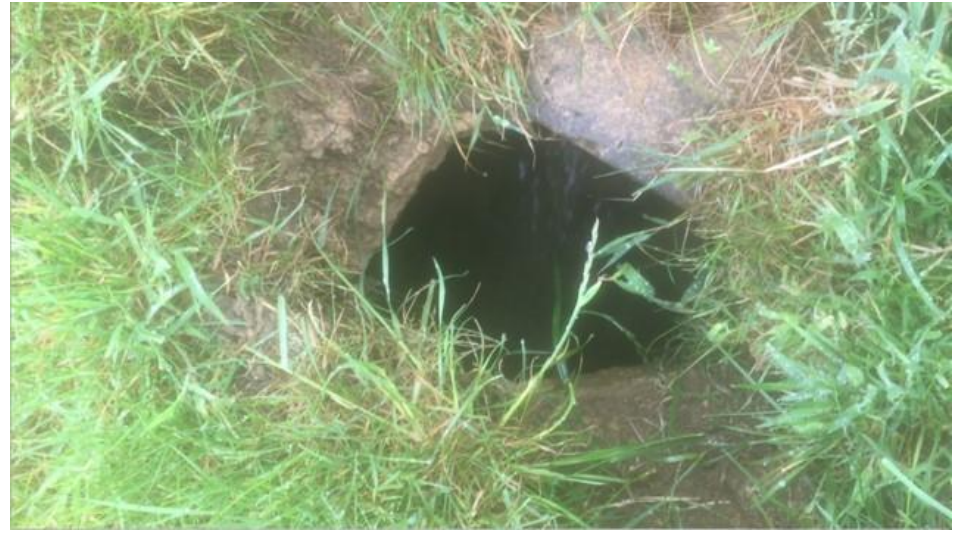
G79_culvert exposed in ground flowing S possible road drainage
