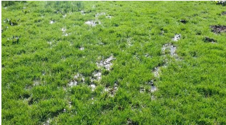
G40_seepage upgradient of River Churn trib starts facing N
