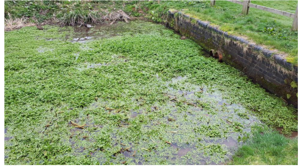
96_looking SE catchpit of flows from NSC
