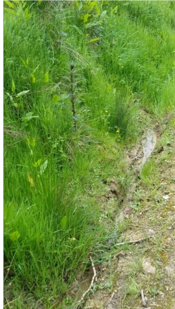
G60_seepages on slope facing S
