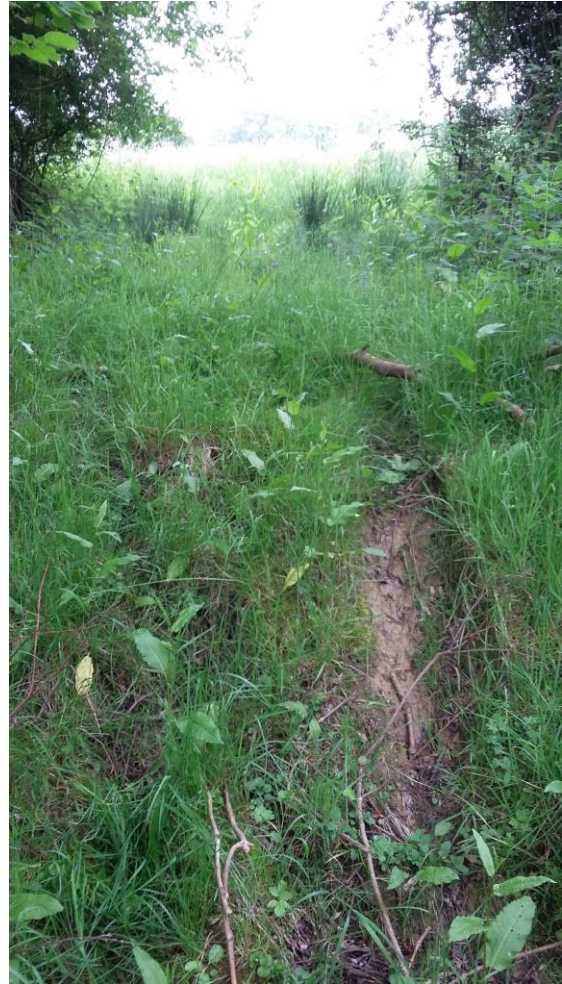
G59_rushes and seepage facing S
