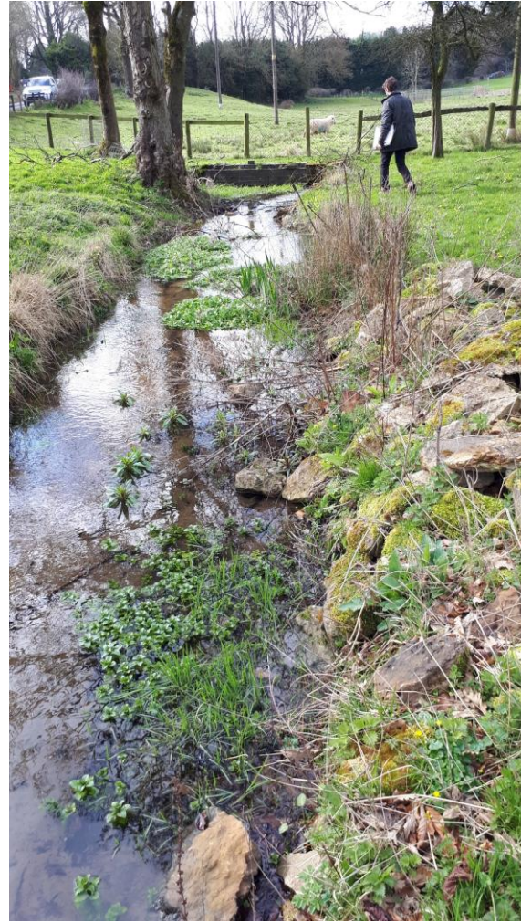
93_looking US of culvert and outfall, showing outfall of flows from golf course, college and seepages
