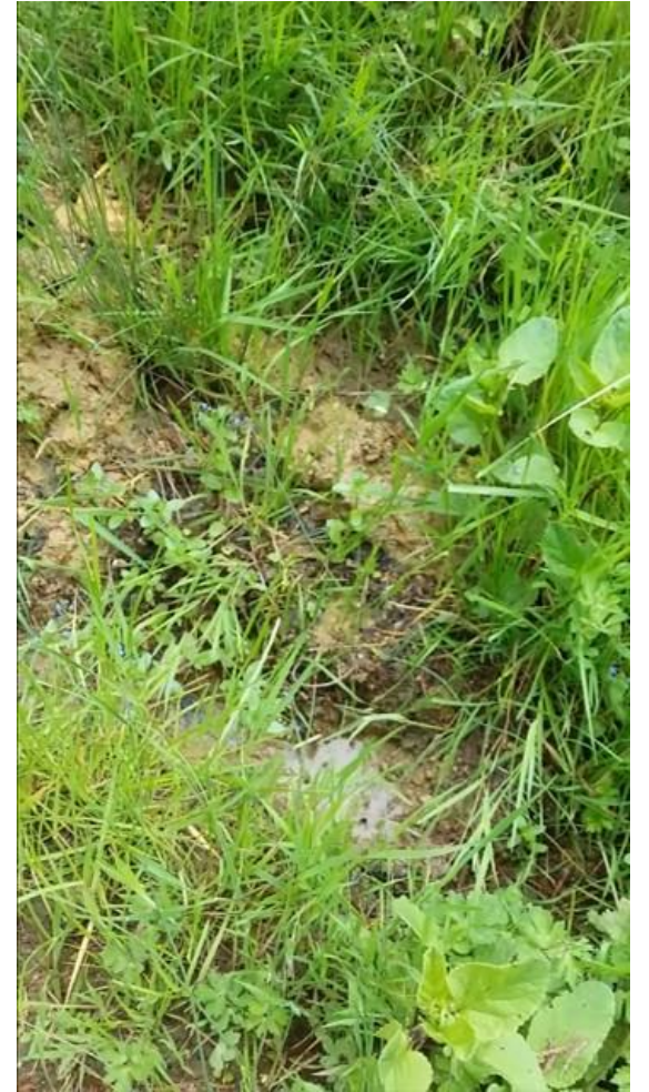
G61_seepage on slope facing S
