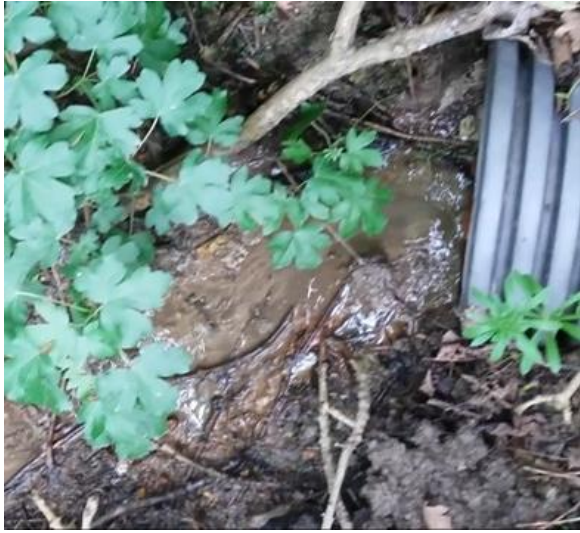
G58_spring fed watercourse culverted under road facing S
