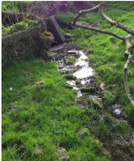
G5_spring_culvert discharge_looking NW
