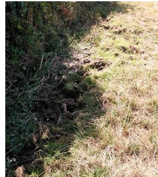
G120_land drain facing E
