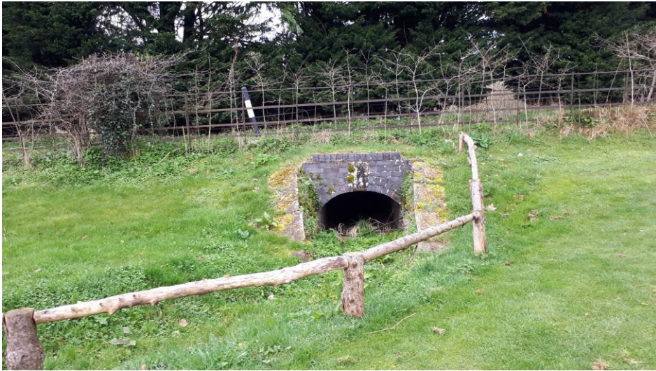
97_looking E US at outfall from national star college
