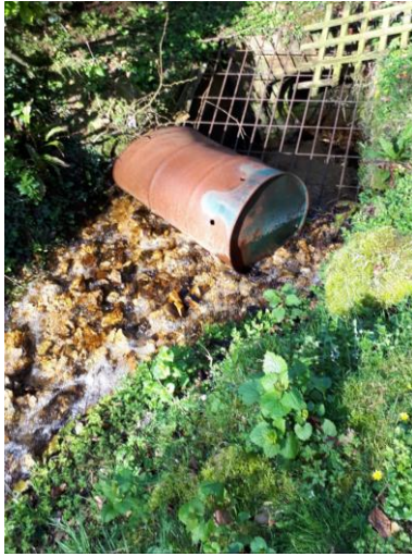
19_looking W DS to culvert under the house_180418
