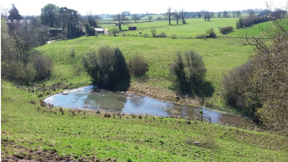
G48_weir and seepage slopes facing S
